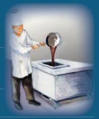
Grease traps servicing restaurant operations should be maintained by regularly cleaning and properly removing grease from the traps. Use of chemical degreasers should be limited as they cause treatment problems at small wastewater treatment plants. All grease should be disposed using a permitted waste hauler.
