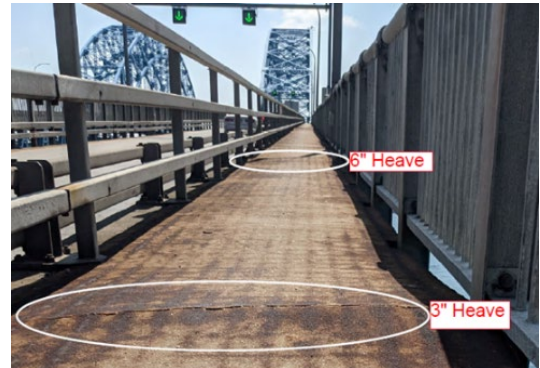
Sidewalk on southbound structure: currently closed due to concrete heaving
