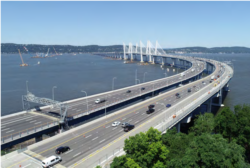
Figure 6: New NY Bridge Project
