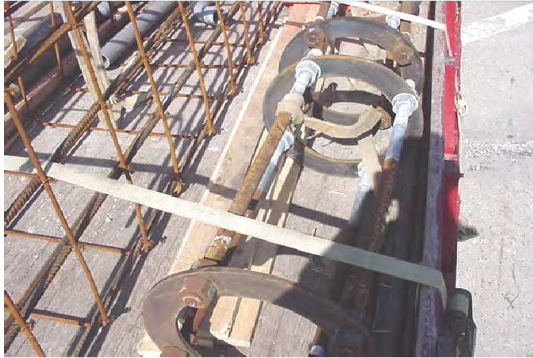
Figure 1. Four Anchor Rod Group in a Template.
