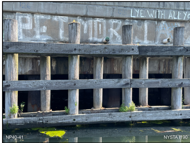
EXISTING TIMBER FENDER SYSTEM
