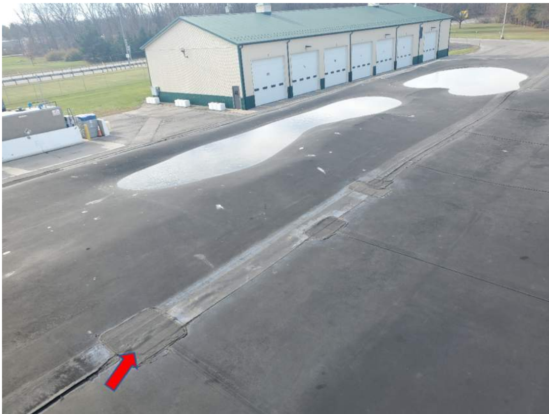
Photograph 19 – View of Roof 3 non-ACM Black Patching Sealant Material (ACM-44, ACM-45 & ACM-46)
