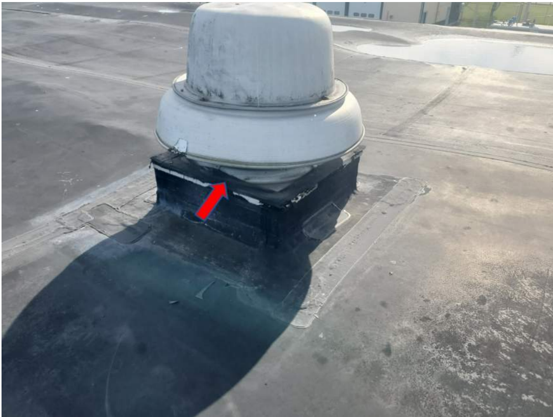
Photograph 15 – View of Roof 3 non-ACM Fan Housing Black Sealant (ACM-34 & ACM-35)
