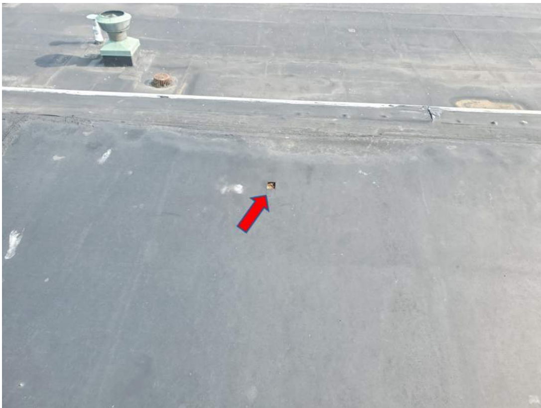
Photograph 21 – View of roof non-ACM Black Fibrous Backing with Tan Foam Material (ACM-50, ACM-51 & ACM-52)
