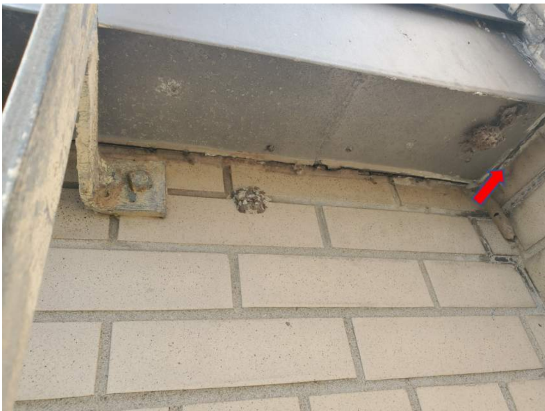
Photograph 22 – View of Roof 3 ACM Overhang of Roof 1 Grey Fibrous Caulk (ACM-53 & ACM-54)
