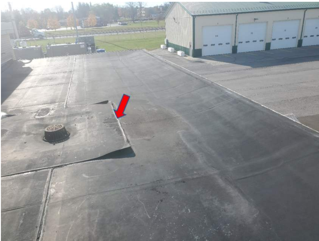
Photograph 7 – View of Roof 7 non-ACM Black Sealant Material from Roof Drain Section and Seams (ACM-13, ACM-14, ACM-15 & ACM-16)
