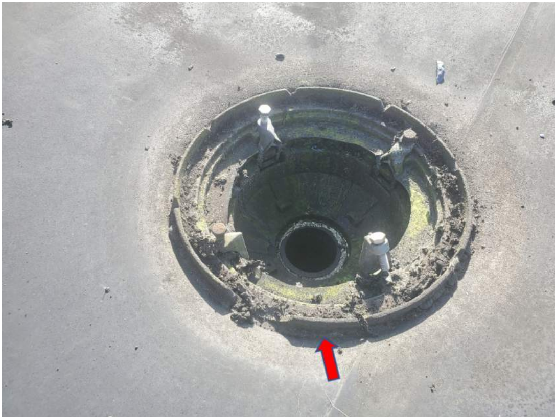
Photograph 9 – View of Roof 7 non-ACM Roof Drain Black Sealant Material (ACM-20 & ACM-21)
