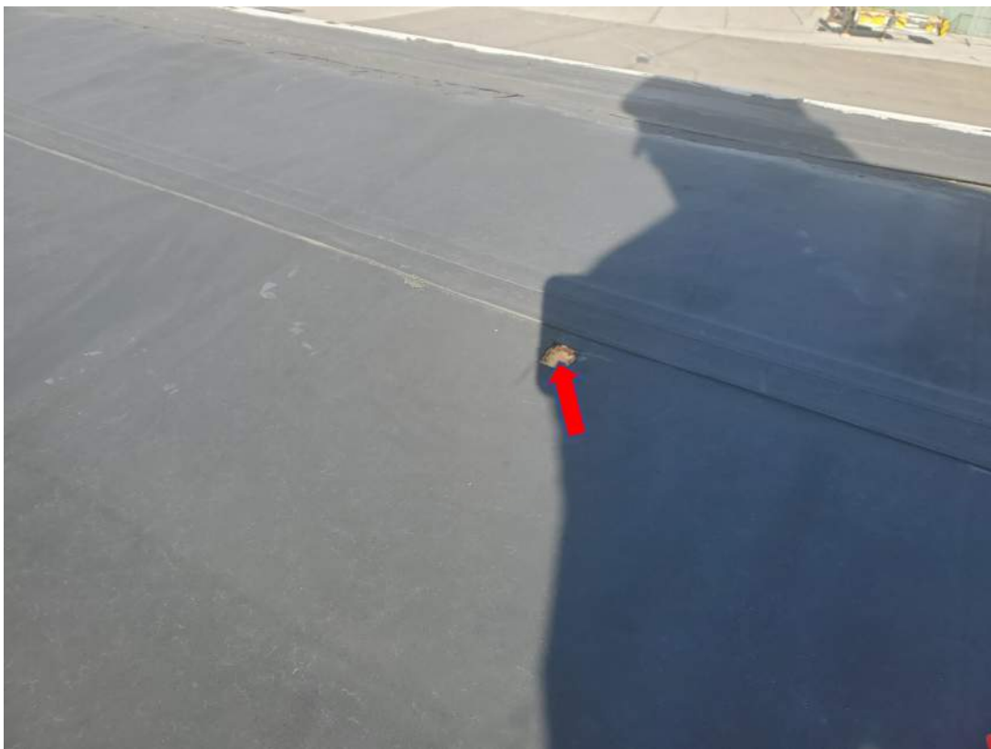
Photograph 12 – Roof 7 non-ACM Black Fibrous Backing Material with Tan Foam Material (ACM-26 & ACM-27)
