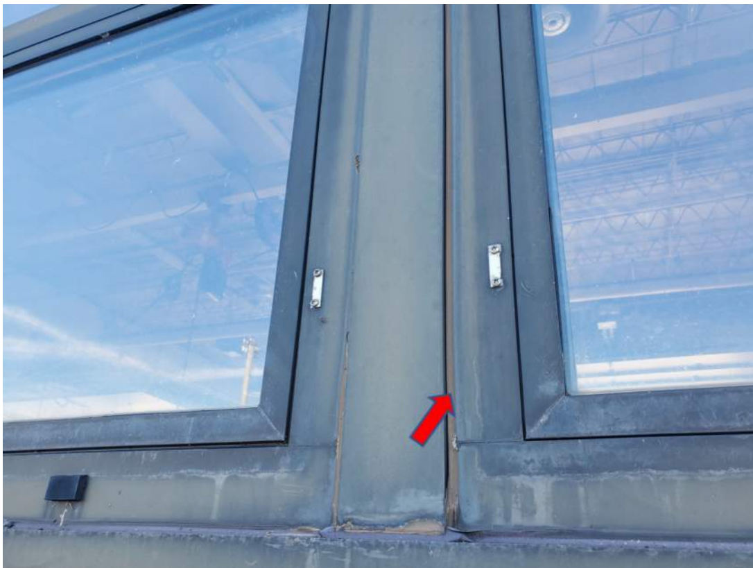
Photograph 27 – View of Garage Exterior non-ACM Brown Window Caulking (ACM-73, ACM-74 & ACM-75)
