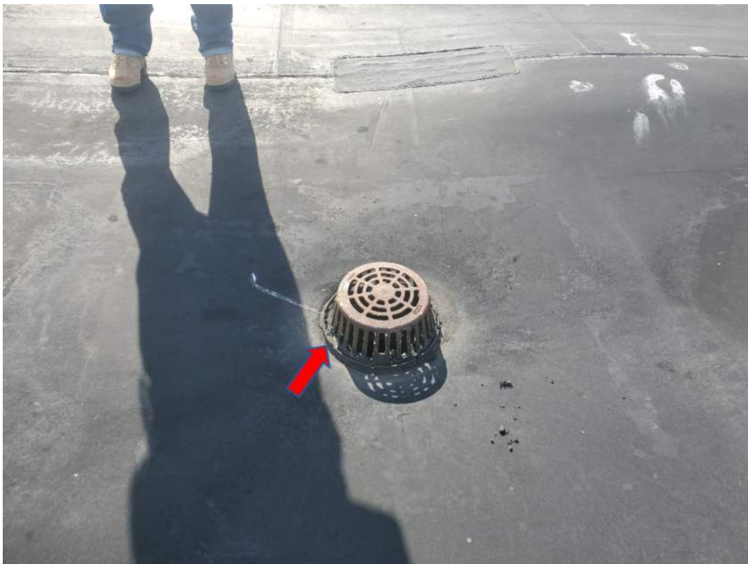
Photograph 17 – View of Roof 3 non-ACM Roof Drain Black Sealant (ACM-40 & ACM-41)
