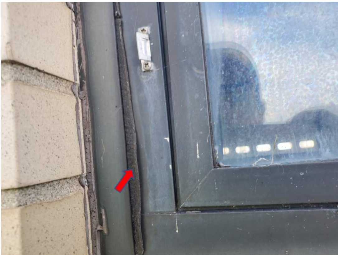
Photograph 25 – View Garage Exterior non-ACM Black Gasket Material (ACM-69 & ACM-70)
