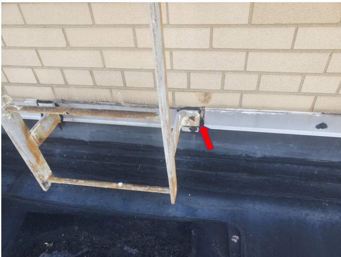
Photograph 2 – View of Roof 7 non-ACM Black Caulking/Sealant on Ladder Bolts (ACM-3 & ACM-4)
