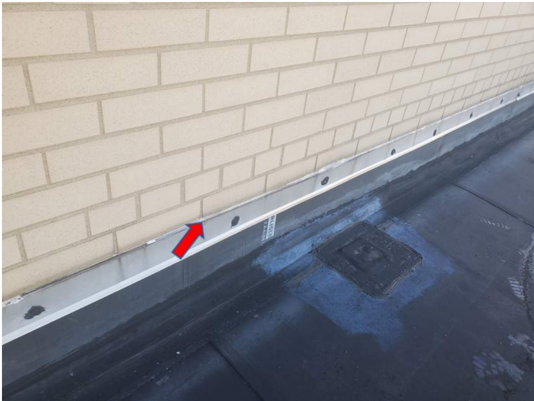
Photograph 3 – View of Roof 7 non-ACM White Caulking on Flashing (ACM-5 & ACM-6)
