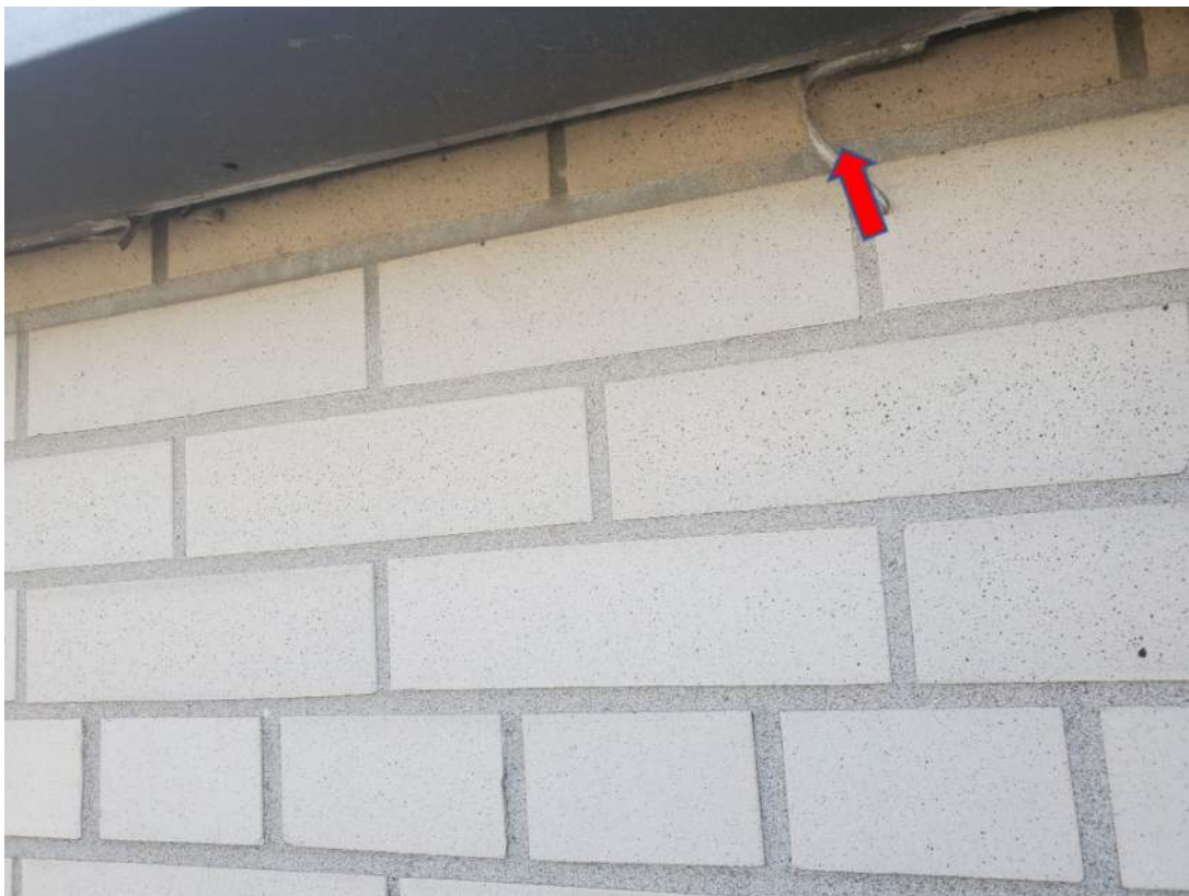
Photograph 5 – View of Roof 3 ACM Grey Fibrous Caulk Underneath Overhang (ACM-9 & ACM-10)
