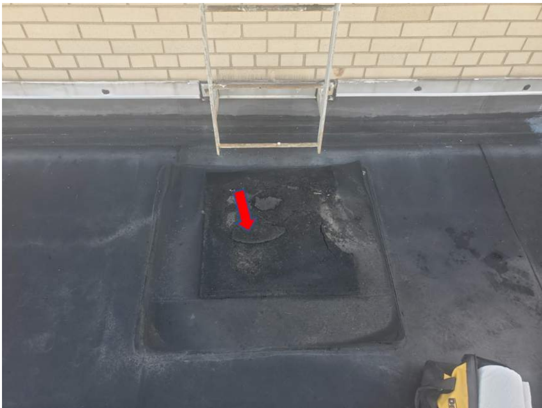
Photograph 1 – View of Roof 7 & Roof 3 non-ACM Black Fibrous Mat Material (ACM-1 & ACM-2)
