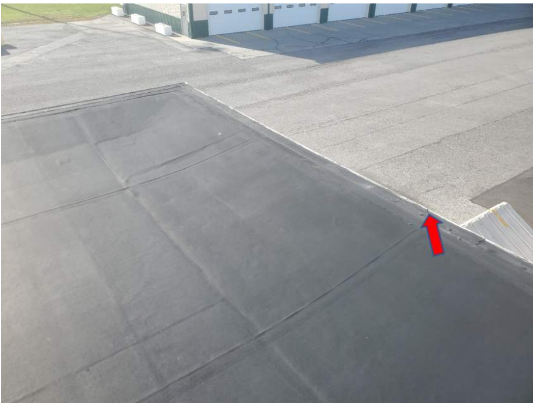
Photograph 8 – View of Roof 7 non-ACM Black Fibrous Caulk/Sealant from Roof Edge (ACM-17, ACM-18 & ACM-19)
