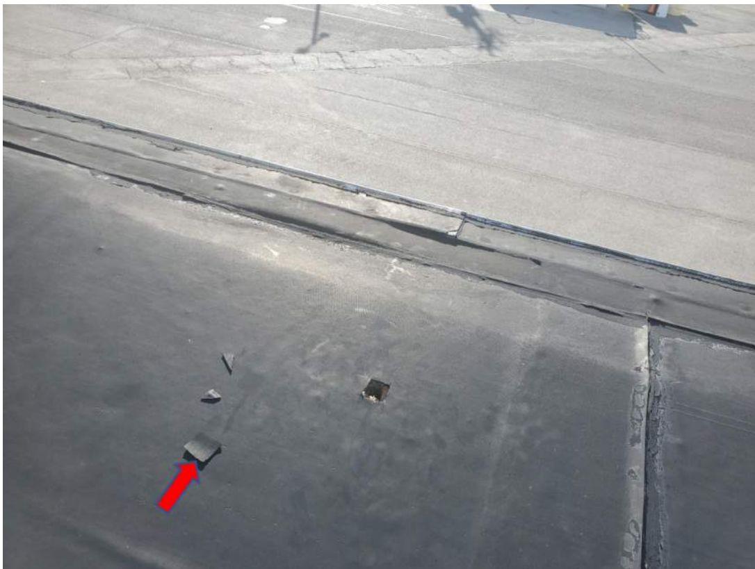
Photograph 11 – View of Roof 7 non-ACM Black Roof Membrane with Fibrous Backing Material (ACM-24 & ACM-25)
