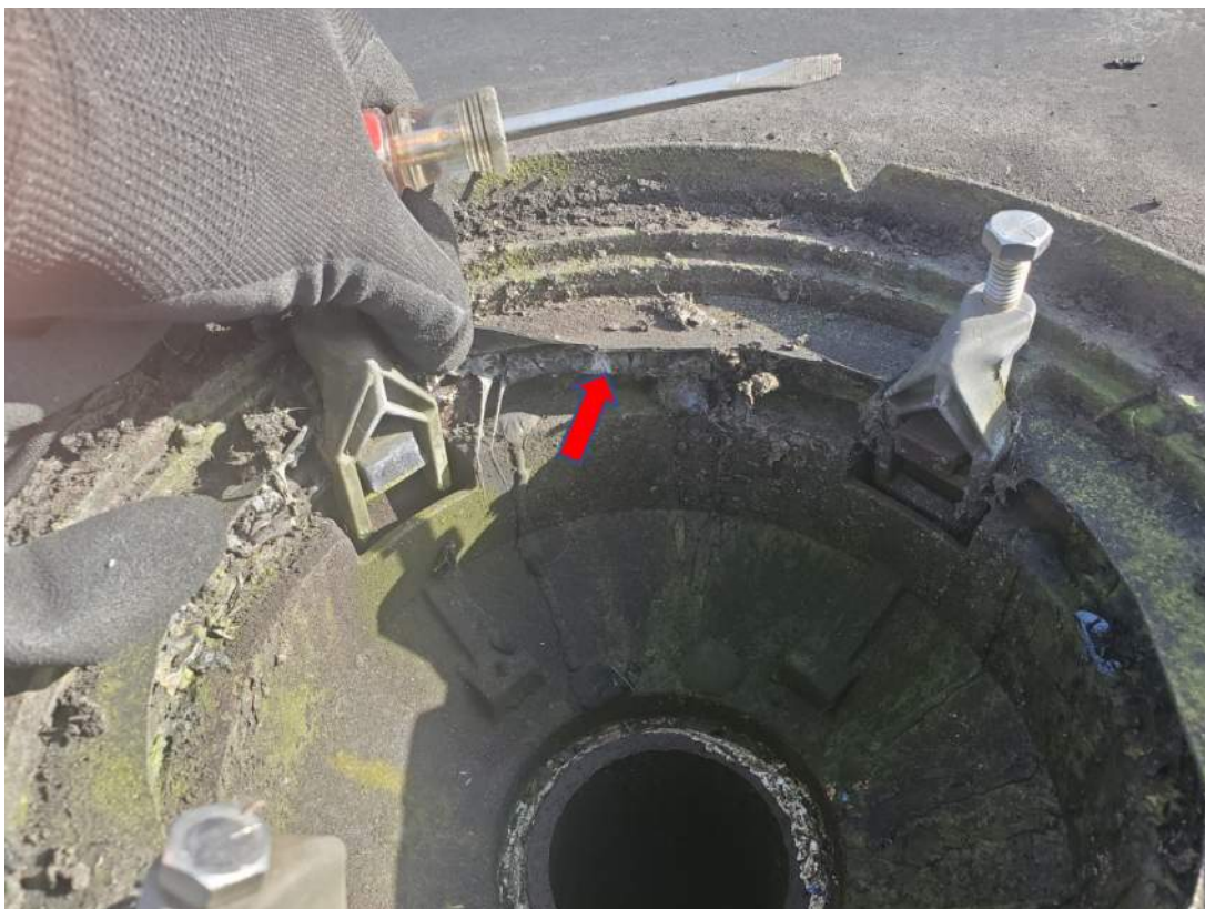
Photograph 10 – View of Roof 7 Roof Drain non-ACM Roof Drain White Sealant material Between Roof Membrane and Underlayment (ACM-22 & ACM-23)
