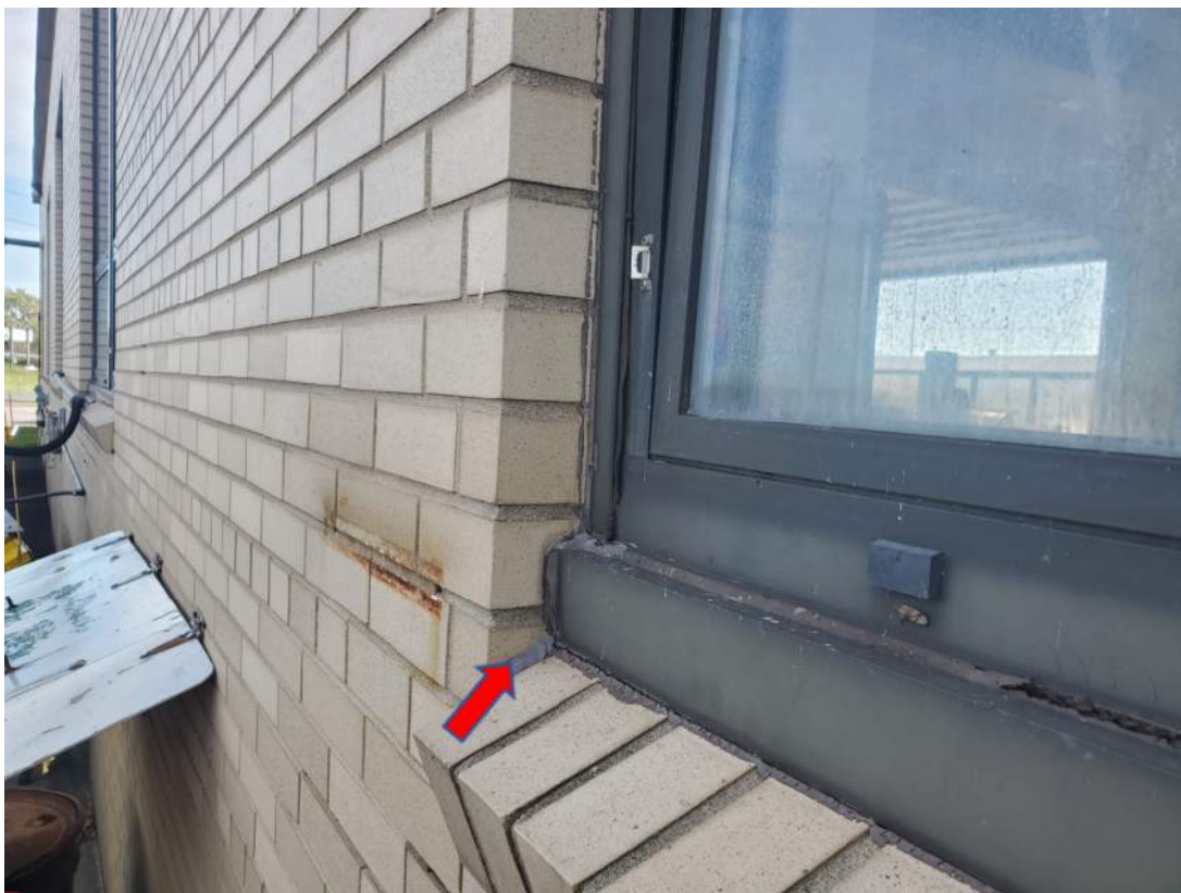
Photograph 26 – View of Garage Exterior non-ACM Light Grey Window Caulking (ACM-71 & ACM-72)
