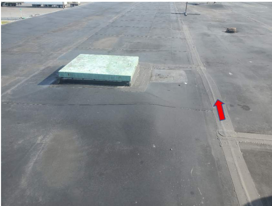
Photograph 16 – View of Roof 3 non-ACM black Seam Sealant Material (ACM-36, ACM-37, ACM-38 & ACM-39)
