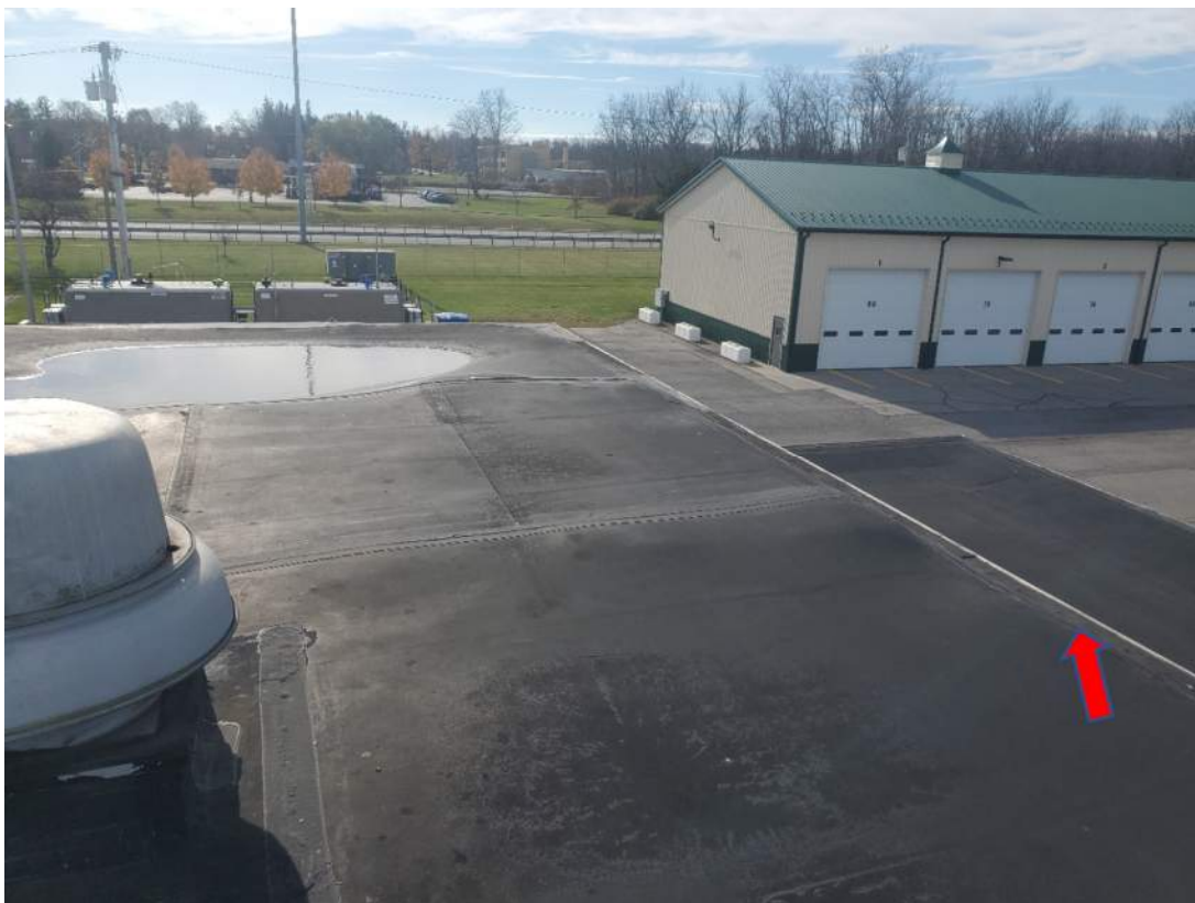
Photograph 14 – View of Roof 3 non-ACM Black Edge Sealant (ACM-30, ACM-31, ACM-32 & ACM-33)
