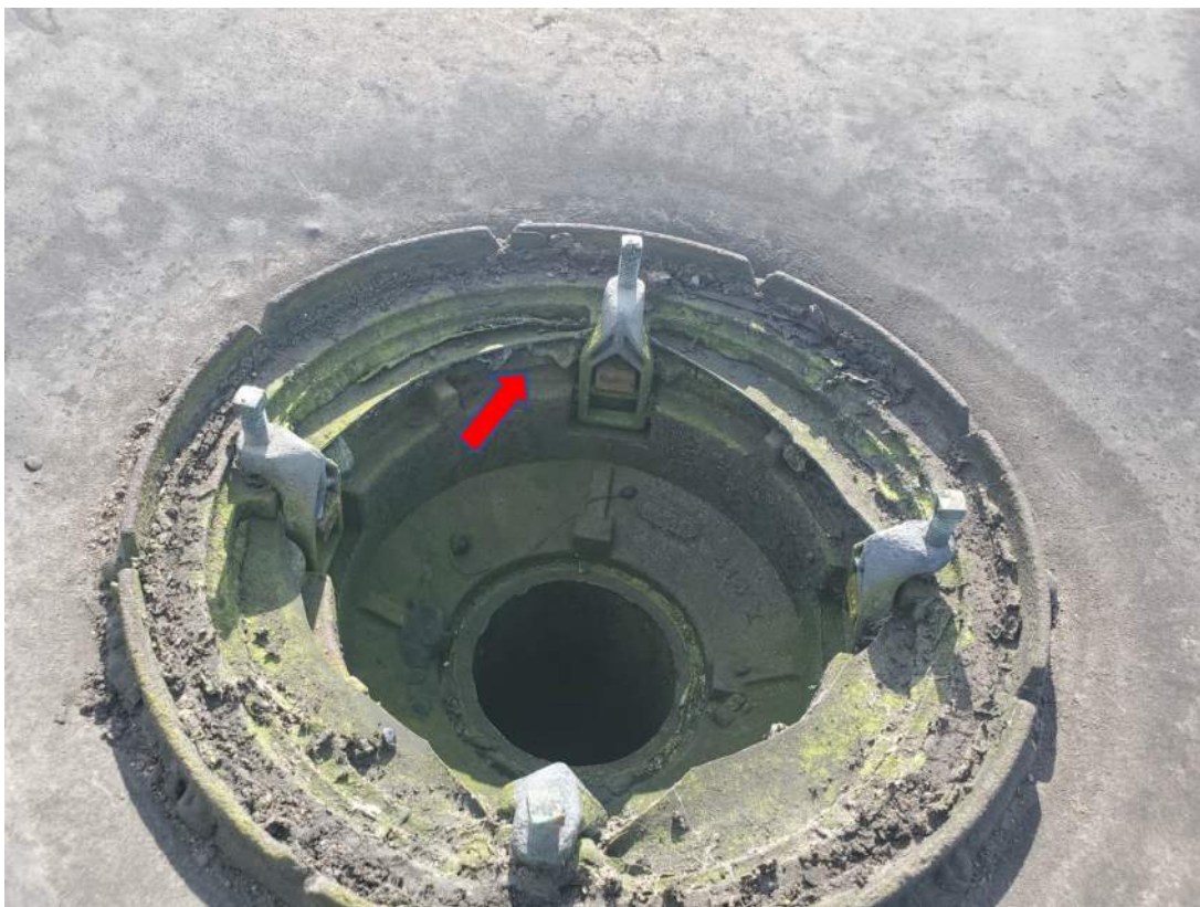
Photograph 18 – View of Roof 3 non-ACM Roof Drain Grey Sealant Between Roof Membrane and Underlayment (ACM-42 & ACM-43)
