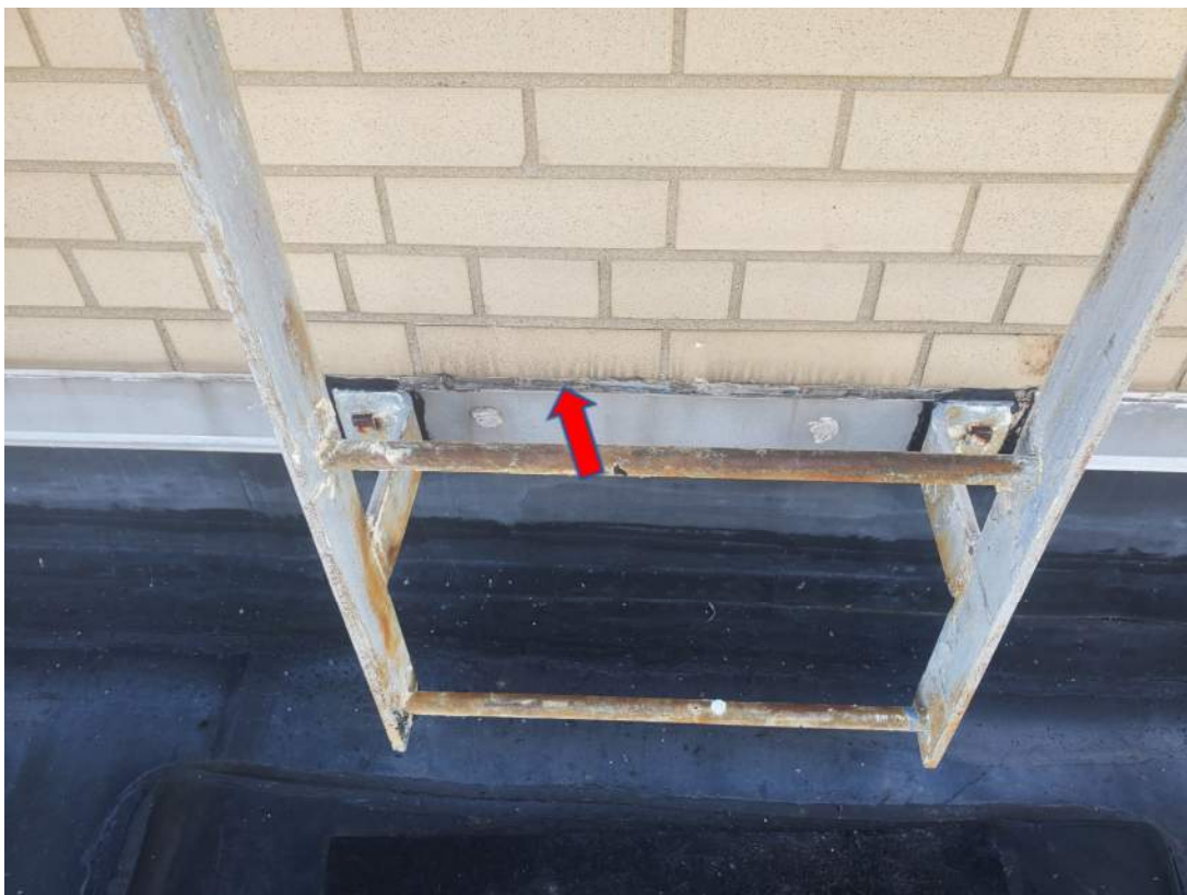
Photograph 4 – View of Roof 7 non-ACM Light Black Caulk Behind Ladder on Flashing (ACM-7 & ACM-8)
