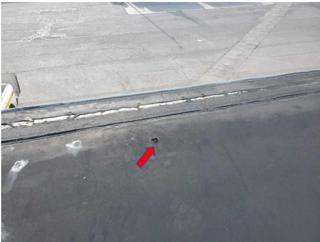
Photograph 20 – View of Roof 3 non-ACM Black Roof Membrane with Fibrous Black Backing Material (ACM-47, ACM-48 & ACM-49)
