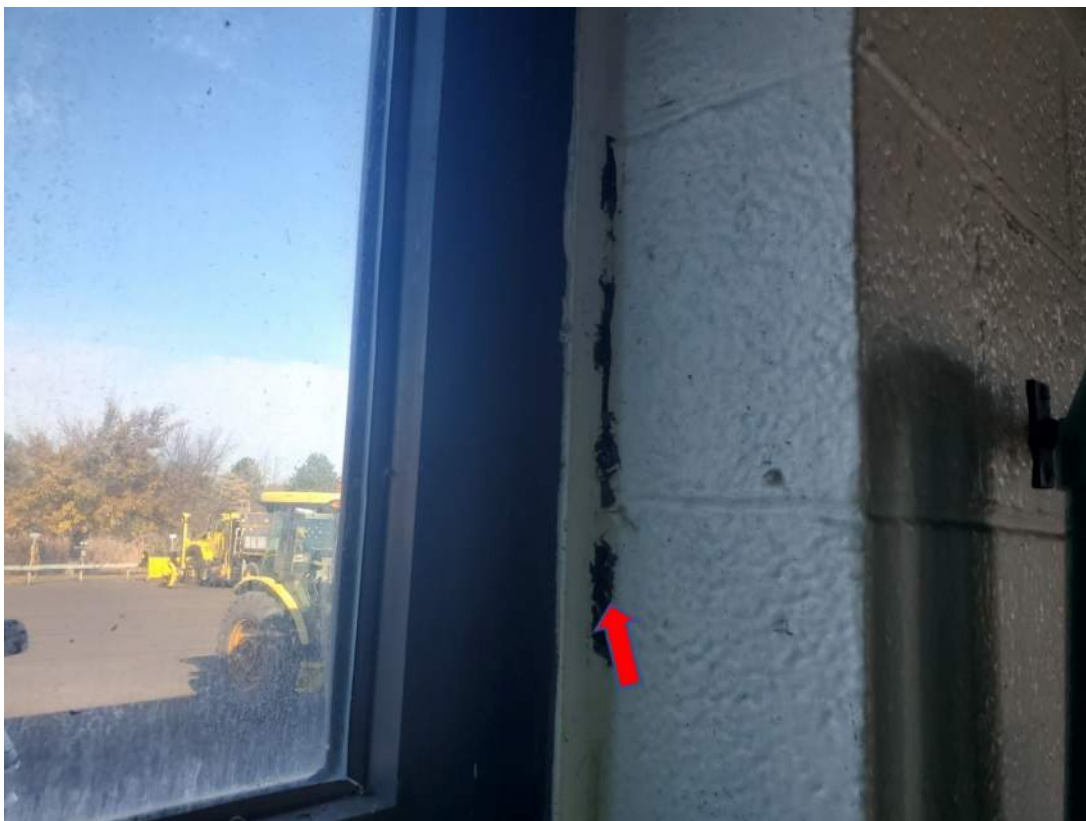
Photograph 28 – View of Garage Interior non-ACM Black Window Caulking (ACM-76, ACM-77 & ACM-78)
