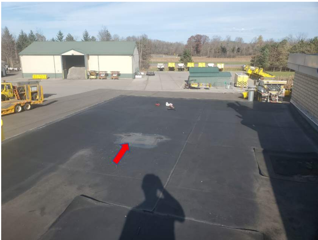
Photograph 13 – View of Roof 7 non-ACM New Black Patching Sealant Material (ACM-28 & ACM-29)
