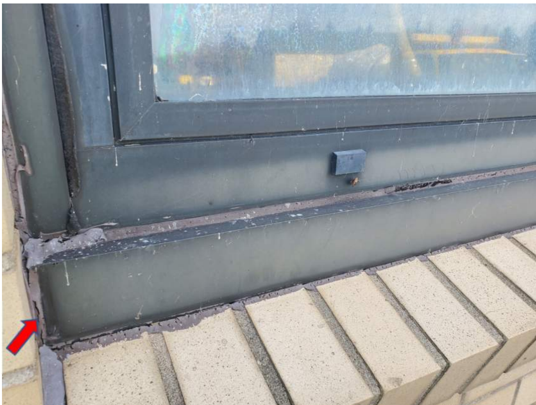
Photograph 24 – View of Garage Exterior non-ACM Light Black Window Framing Caulk (ACM-66, ACM-67 & ACM-68)
