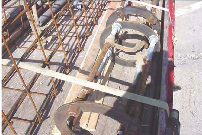
Figure 1. Four Anchor Rod Group in a Template.
