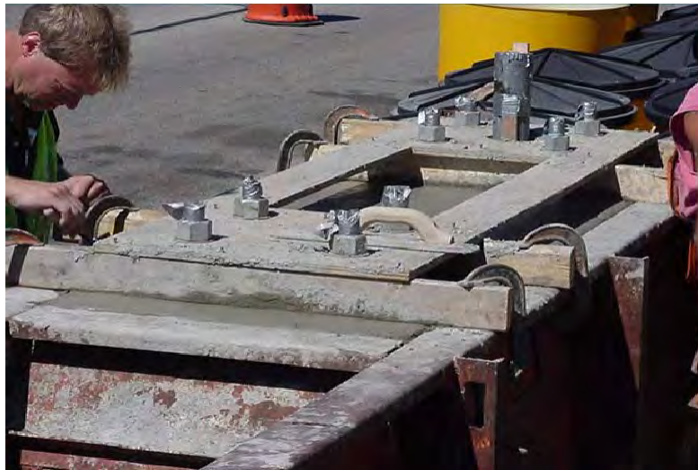
Figure 2. Template Secured to the Forms to Ensure Proper Alignment. Note Anchor Rod Threads Taped to Prevent Contamination by Concrete.
