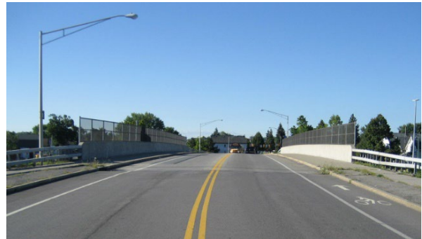
Exhibit 3: Bridges over I-190 provide important multi-modal community connections (Ogden Street Bridge).
