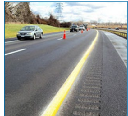
Exhibit 11: Recess Triple Drop Pavement Markings
