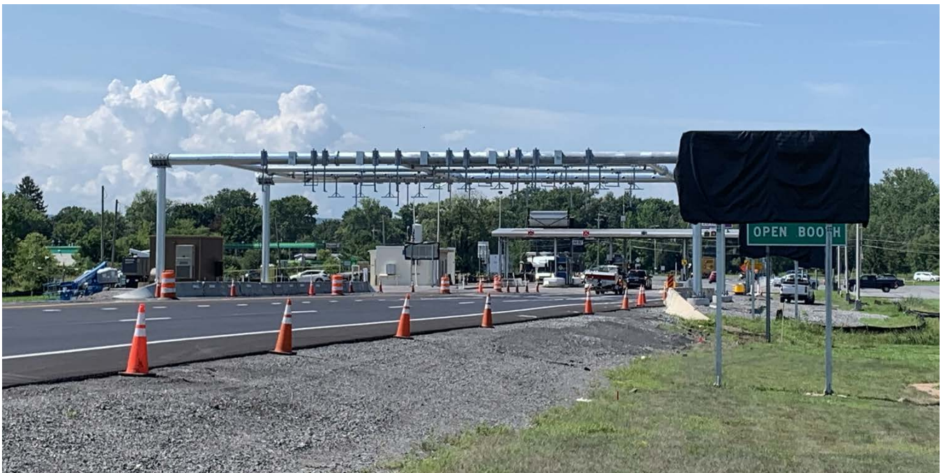
Figure 6: Example of Thruway Cashless Tolling Gantry Before Toll Plaza Removal
